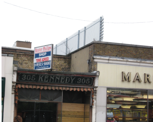
Metal fence detracting from street scene
