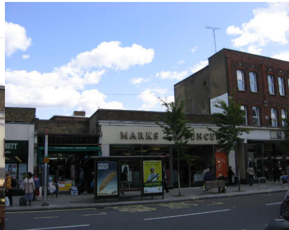
Metal fence removed to the benefit of street scene
